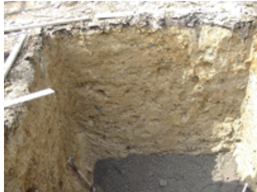
Digging a hole.
